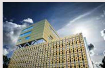
The Nest graces Ulriksdal in Solna with its innovative architecture and decisive presence. It contains the gym chain Actic's headquarters and a top modern gym. The property was completed and acquired by Annehem Fastigheter in 2020.
